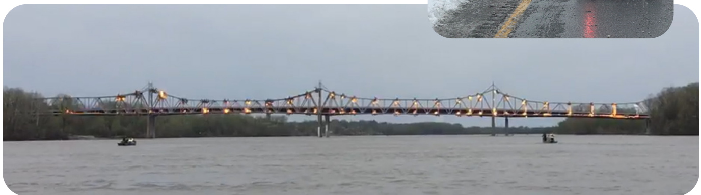
Troopers assisted with the historic bridge implosion of the Missouri River Bridge in Franklin County.
