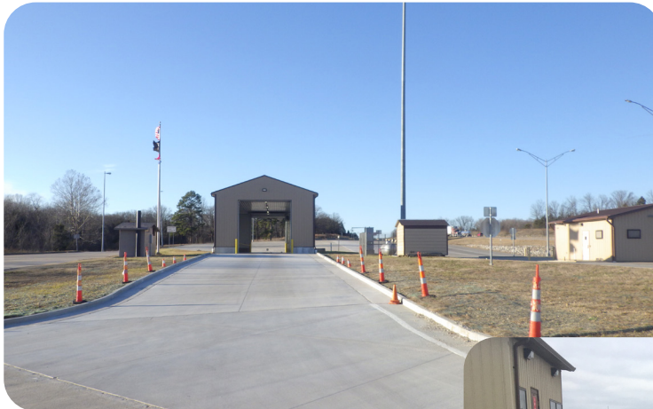
The C5 South inspection building in Bloomsdale, MO, was completed in 2019.
