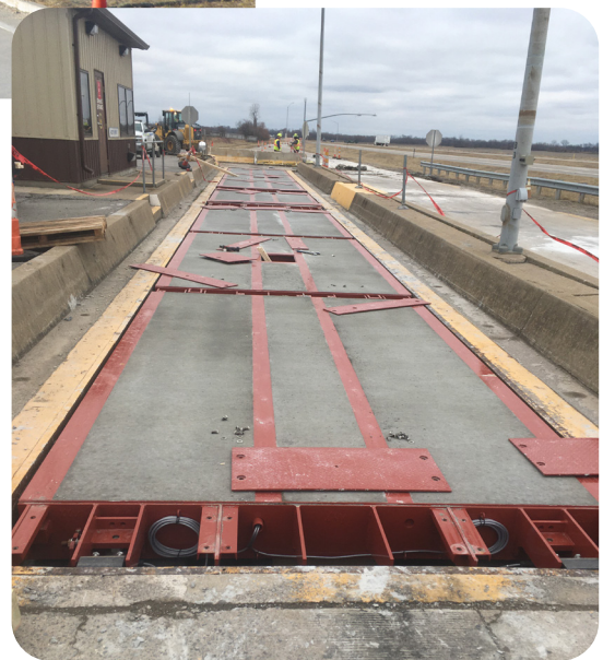
The E1 South platform scale was replaced in 2019.
