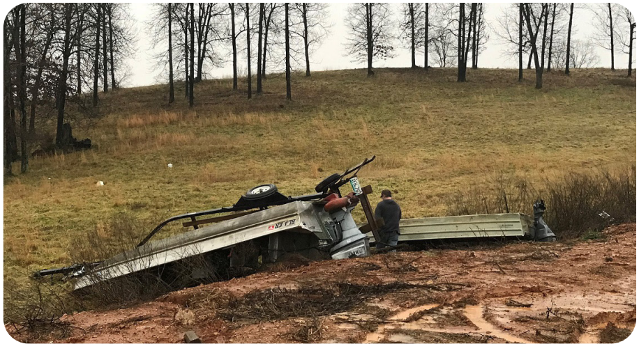
On February 7, 2019, a strong storm tore through the Doniphan area causing serious damage to buildings of a local boat dealership.
